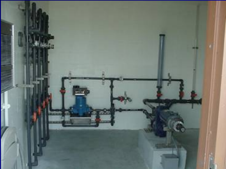
Alum Injection Equipment
