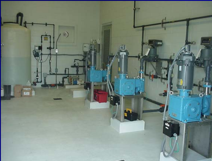
Alum Injection Equipment
