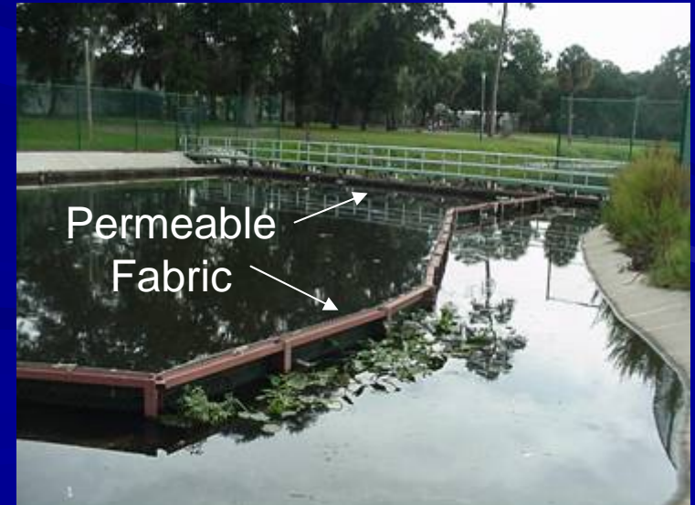
In-line Floc Trap
