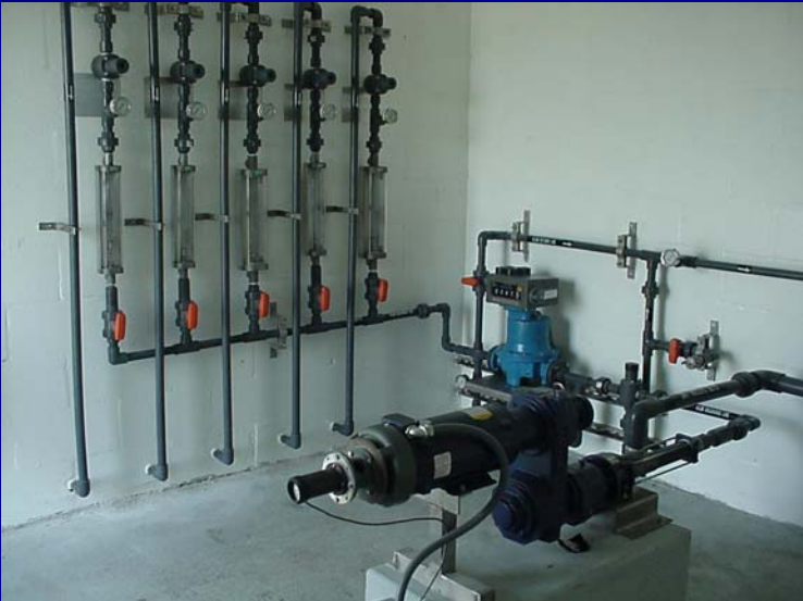
Alum Injection Equipment
