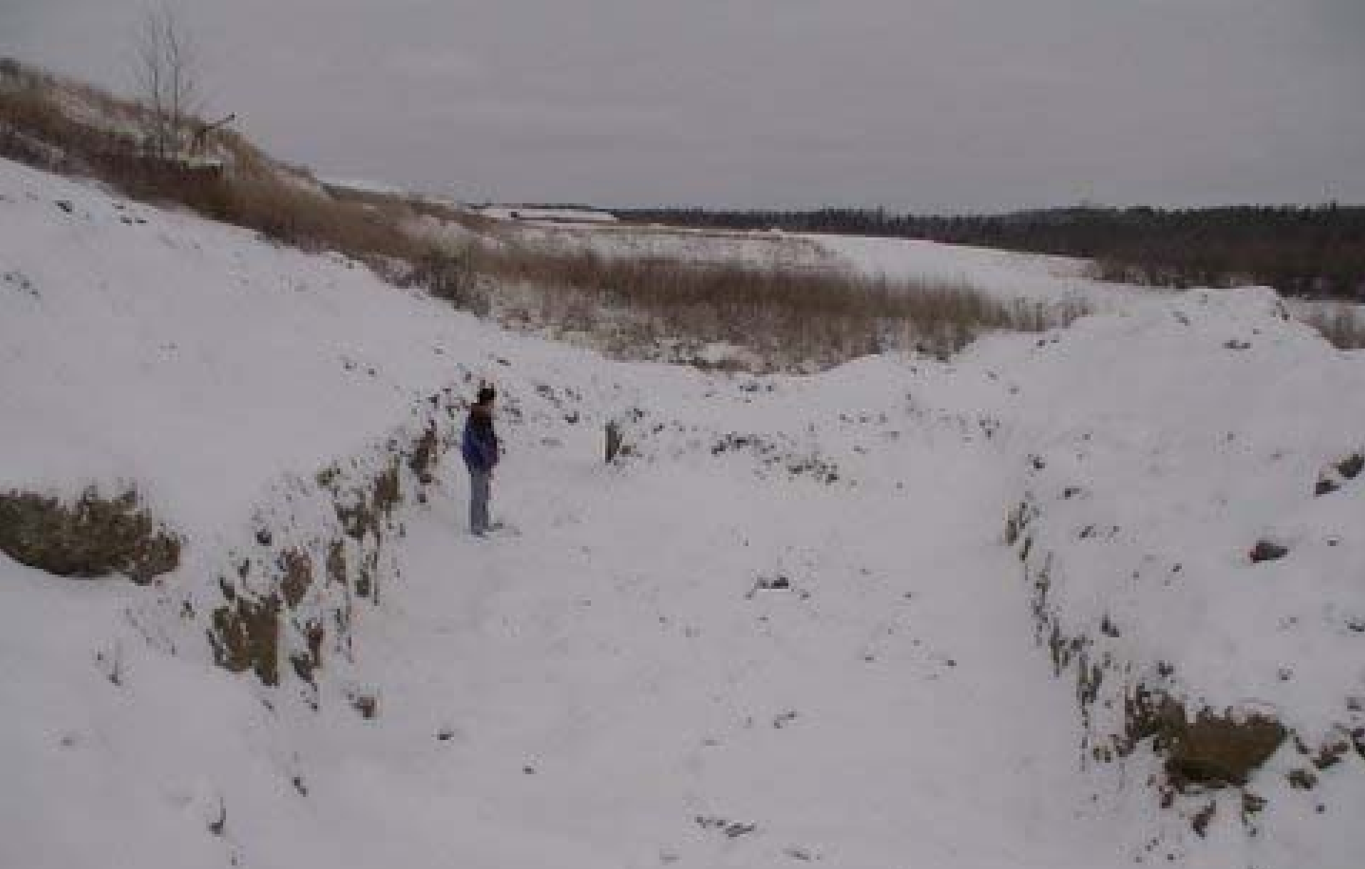
Mixing chamber installation at -15 Celsius
