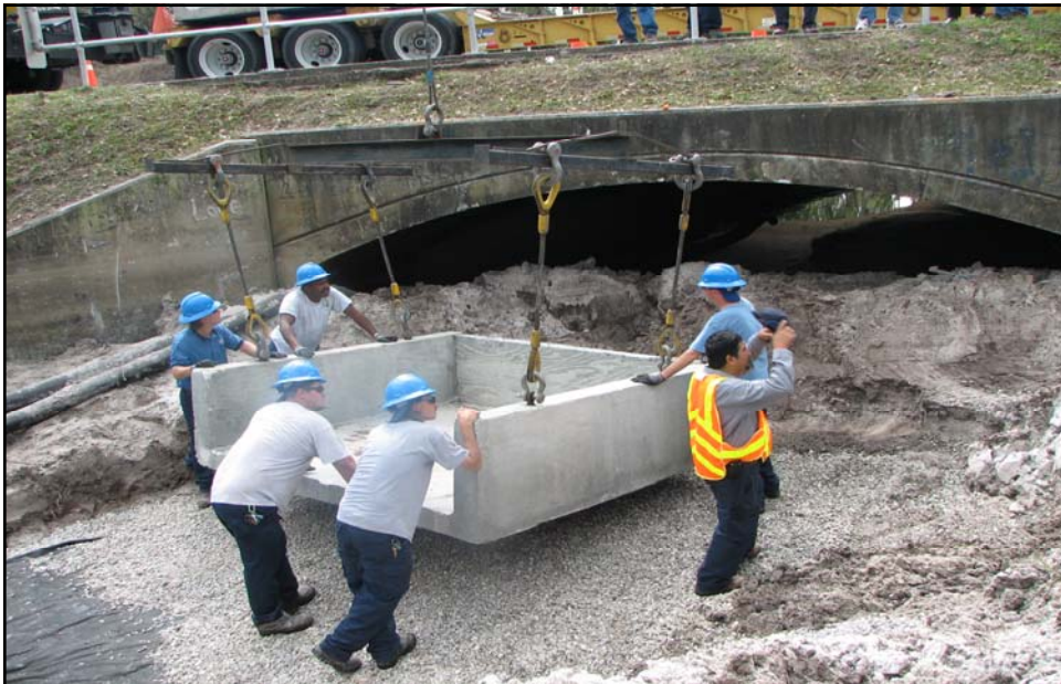
U-CHANNEL INSTALLATION
