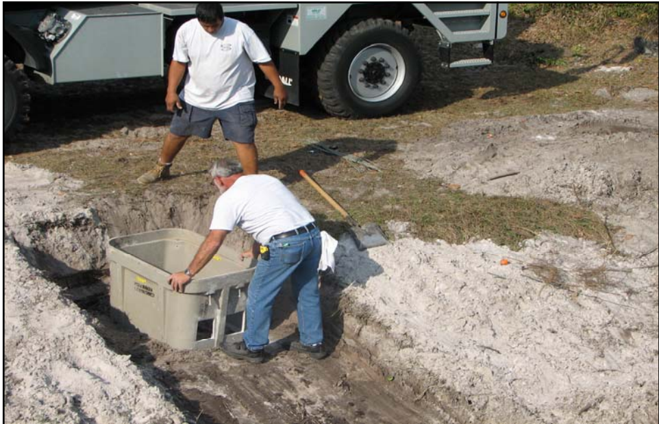
U-CHANNEL INSTALLATION
