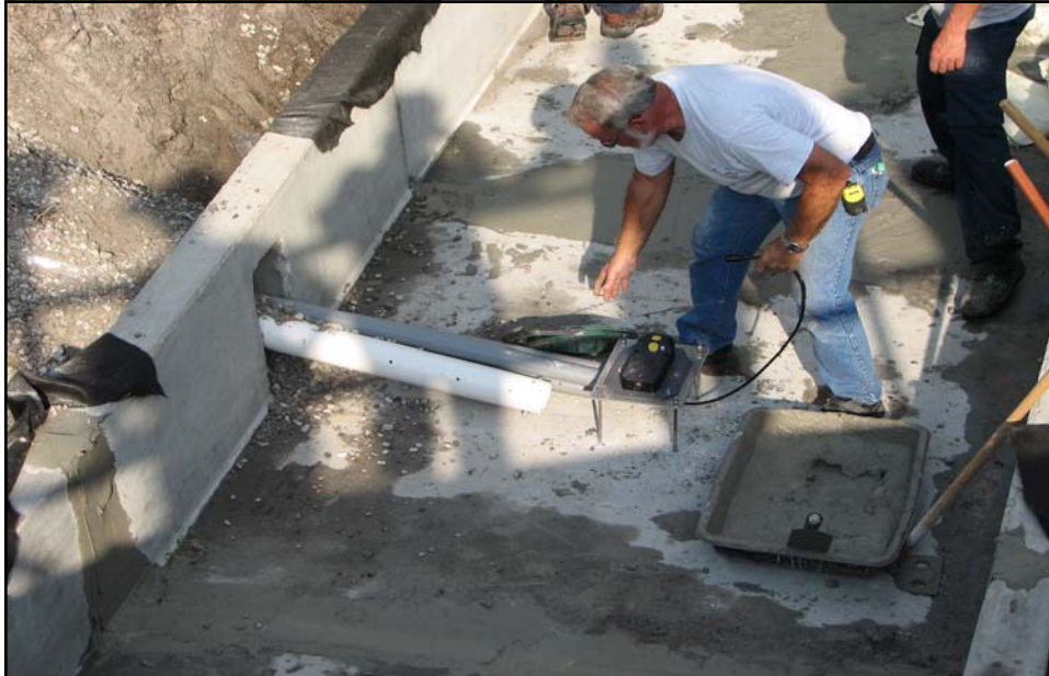
U-CHANNEL INSTALLATION
