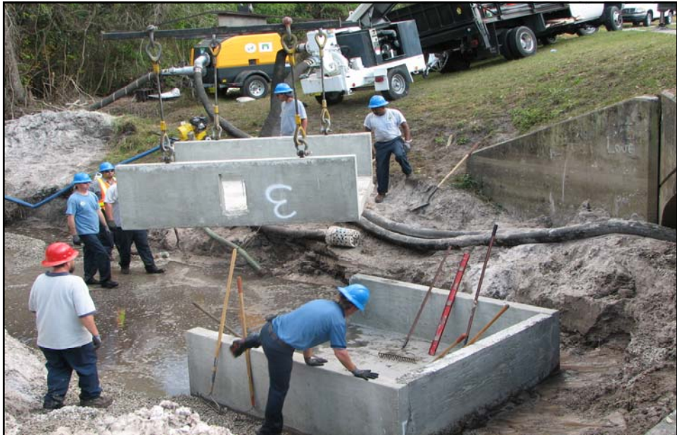
U-CHANNEL INSTALLATION
