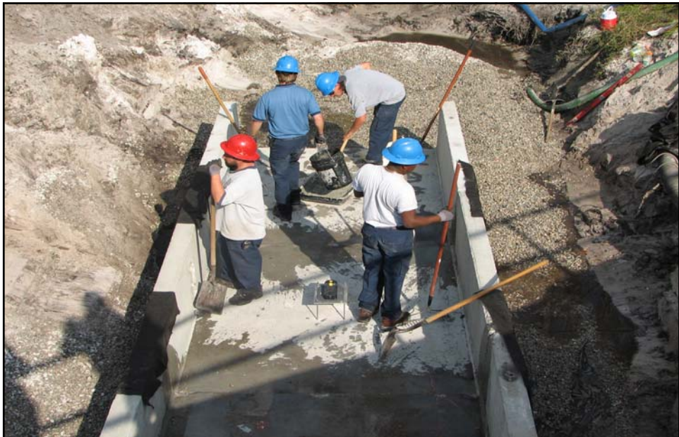
U-CHANNEL INSTALLATION
