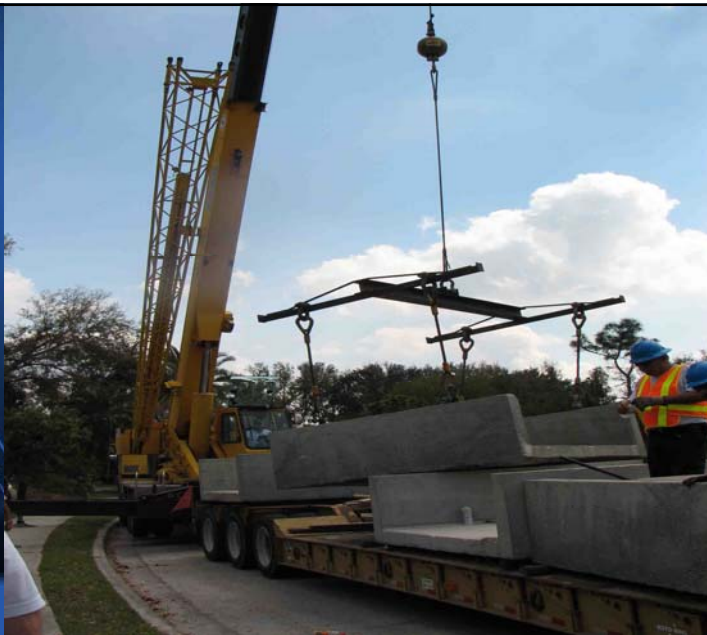
U-CHANNEL INSTALLATION
