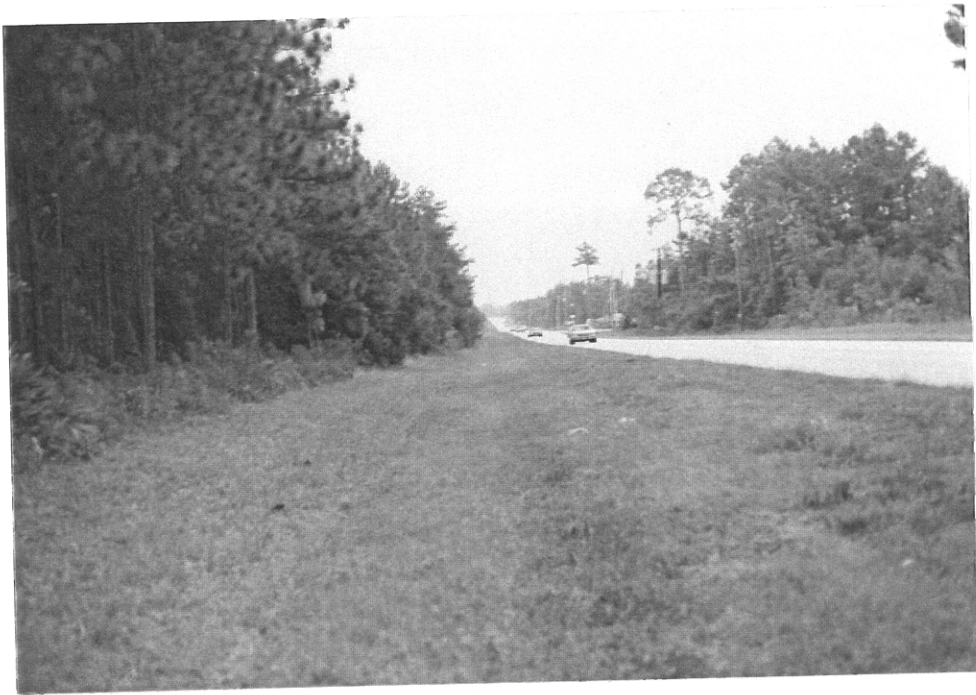
Fig. 23. Swale at SR 520 north of Orange County line (L).
