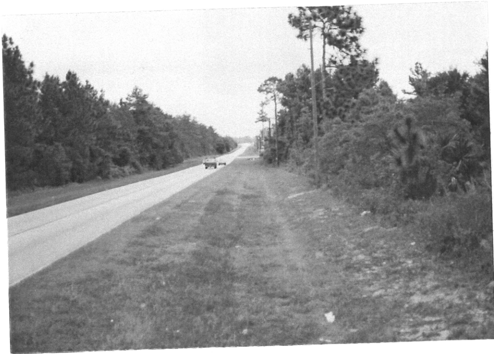
Fig. 24. Swale at SR 520 north of Orange County line (R).
