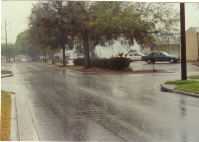
COLLECTS RUNOFF WATER
