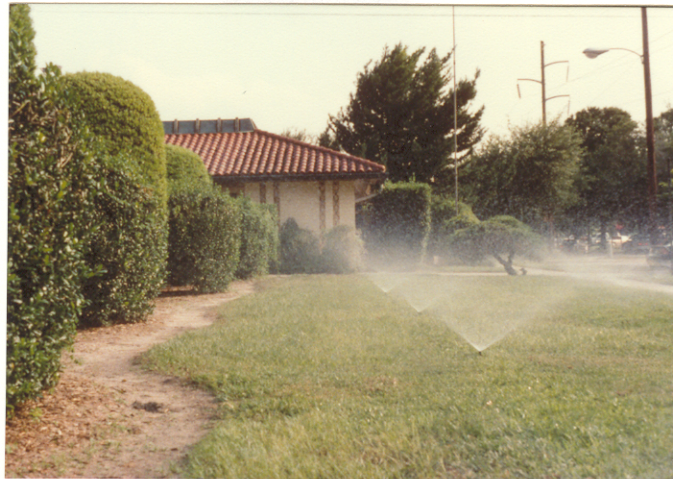
AND REUSES THE WATER
