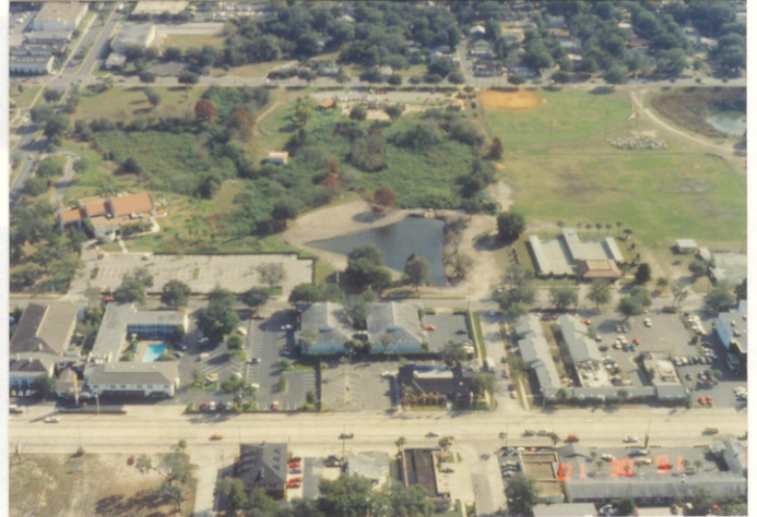
RESTORATION-IN-PROGRESS WATERSHED AREA AND POND
