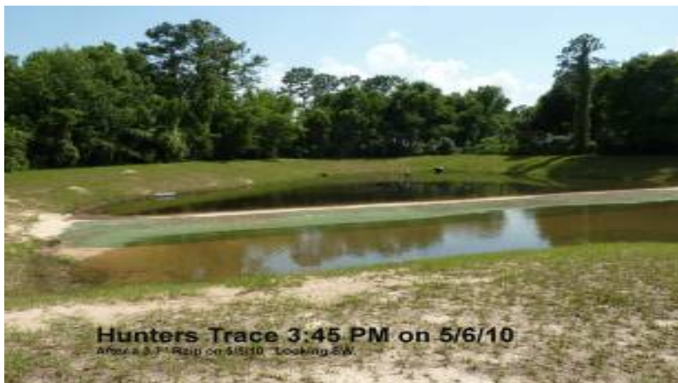
Figure 25 New integrated design at the Hunters Trace basin (Pollution Control Basin is in background; Flood Control Basin is in foreground) after placement of erosion control blanket showing good performance and absence of erosion after 3.7-inch storm.
