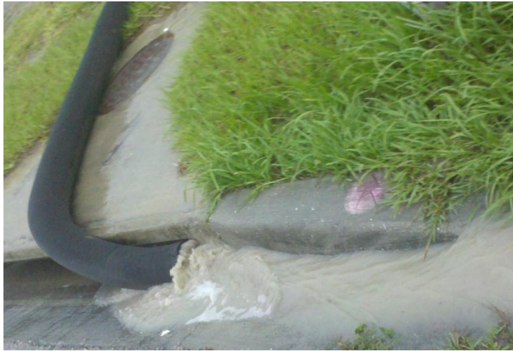
Figure 4: Improper curb inlet protection practice
