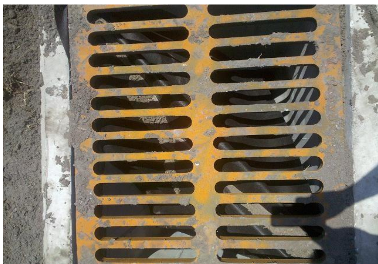
Figure 3: Improper drop inlet protection
