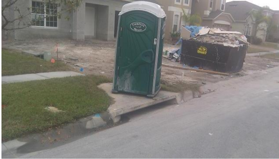
Figure 2: Absence of inlet protection on residential construction
