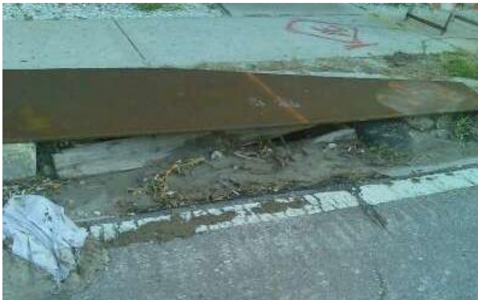
Figure 1: Lack of inlet protection
