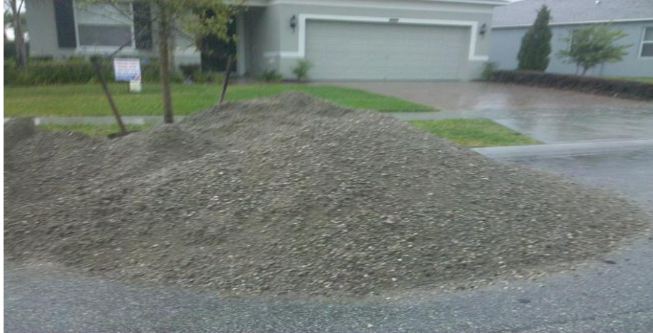
Figure 5: Improper aggregate storage
