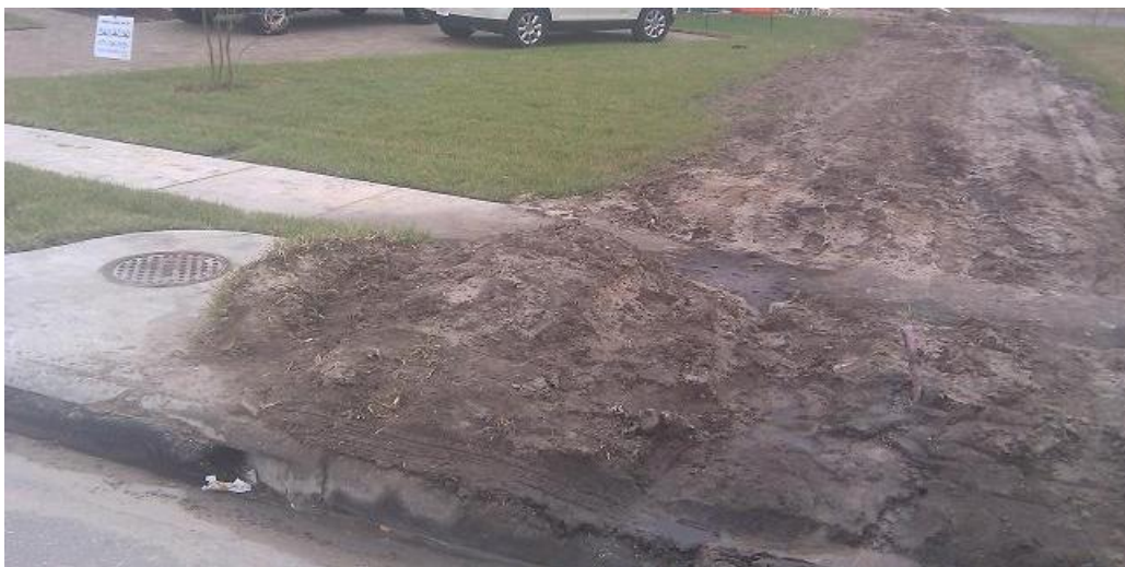
Figure 6: No source control adjacent to inlet
