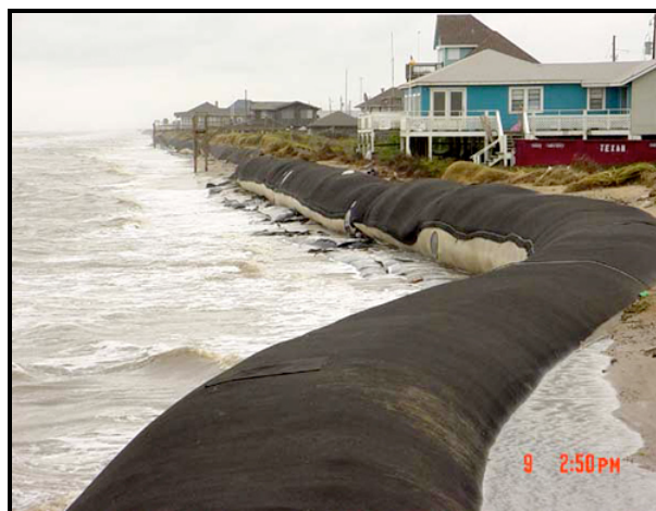
Sandsock, sand-filled tubular geotextile (Source: Surfrider Foundation, 2006)
