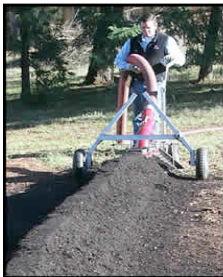
Installation of compost berm (Source: Rexius, 2006)
