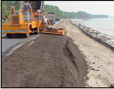
Placement of compost mulch layer
