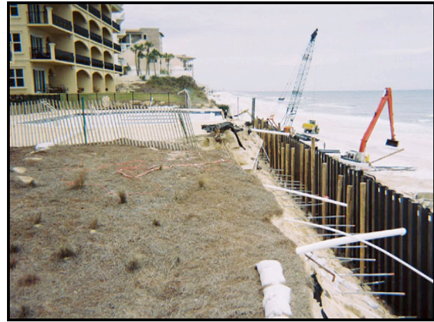
Protection of construction site using sheet-pile barrier and jute fiber mat (Source: Foundation Technologies, 2006)
