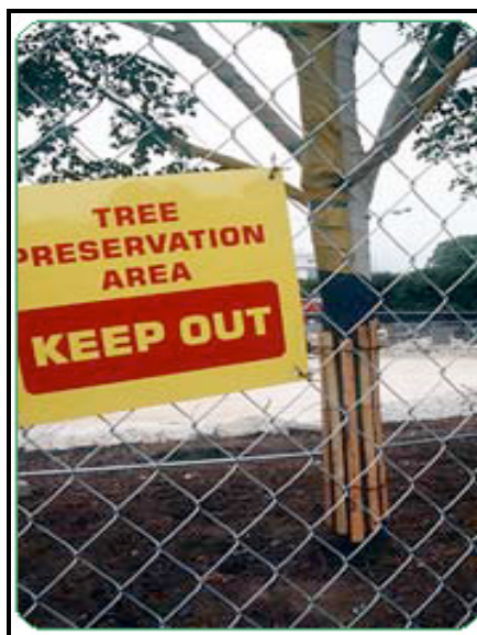
Marked tree preservation area in construction zone (Source: National Gallery, 2006)
