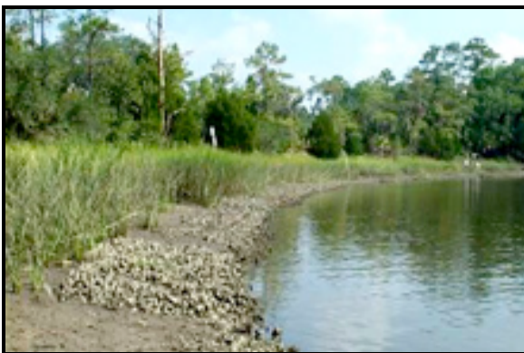
Armoring with oyster habitat and constructed wetlands (Source: NOAA, 2006)
