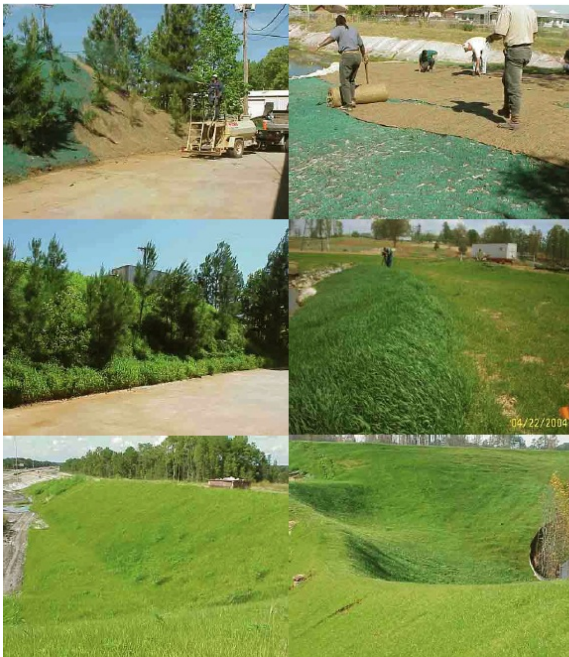
Figure AIII-7: Polymer-enhanced Turf Reinforced Matting.
