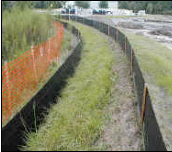
SRB prior to placement of mulch barrier (Source: Florida Dept. of Env. Protection, 1988)
