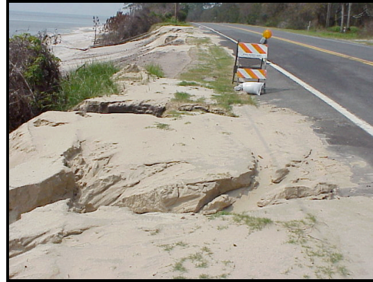
Sheet and gully erosion along shoulder, August 2005
