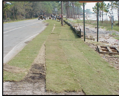
Final placement of sod
