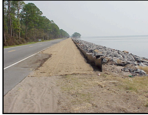
Placement of jute fiber erosion control blanket
