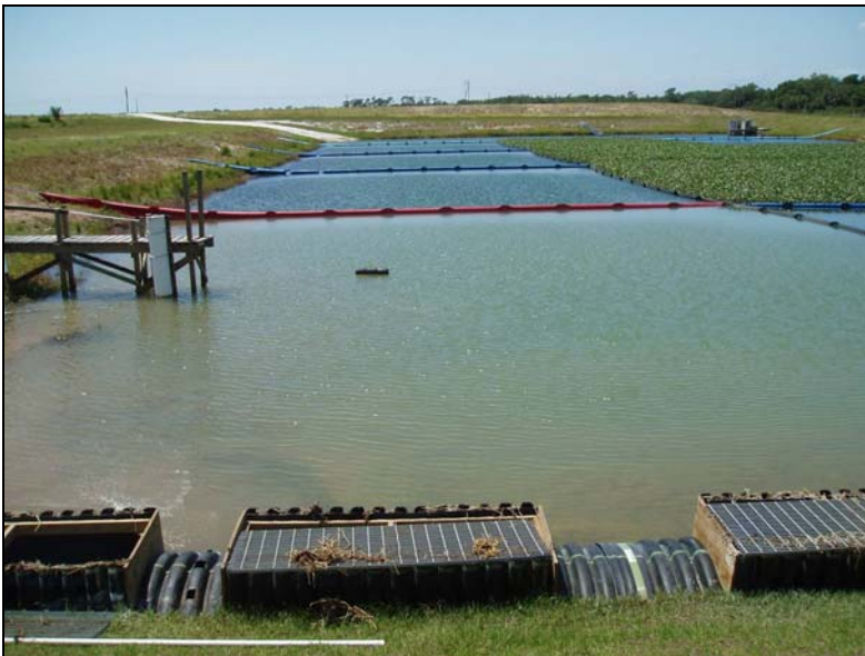
Figure 12. The Nubbin Slough HWTT. The mixing chamber and inflow manifold are in the foreground, and the outflow riser is in the upper right of the photo.
