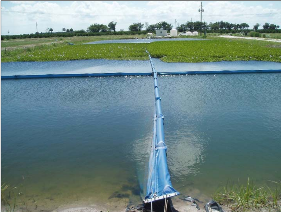
Figure 6. The outflow region of the Ideal Grove HWTT, with the northern (A) flow path on the right, and the southern (B) flow path on the left. The northern flow path receives continuous amendment additions, while the southern flow path receives amendments only intermittently.
