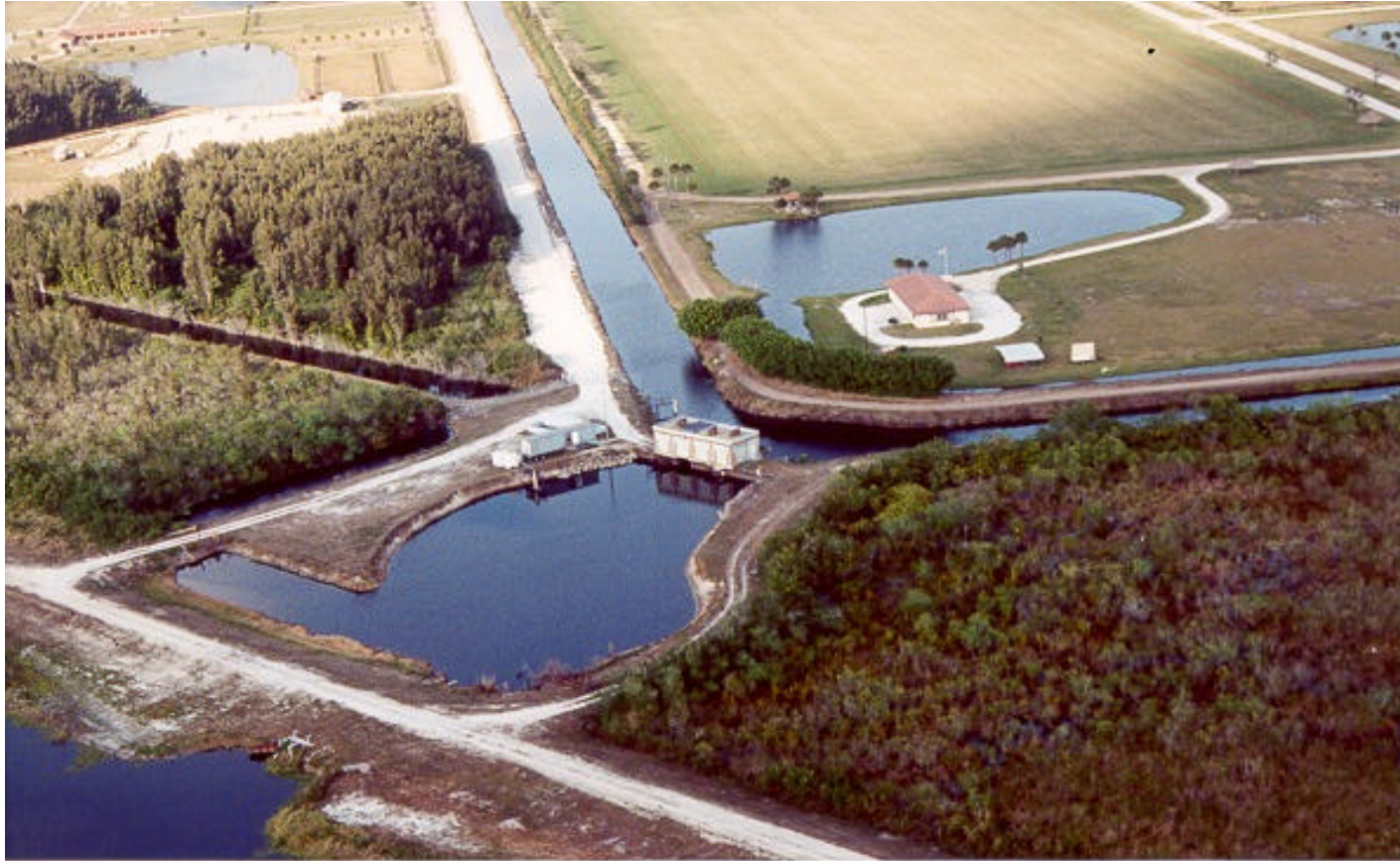
FIGURE 3. CTSS TREATMENT TRAILER at Wellington Pump Station No. 2 (aerial)
