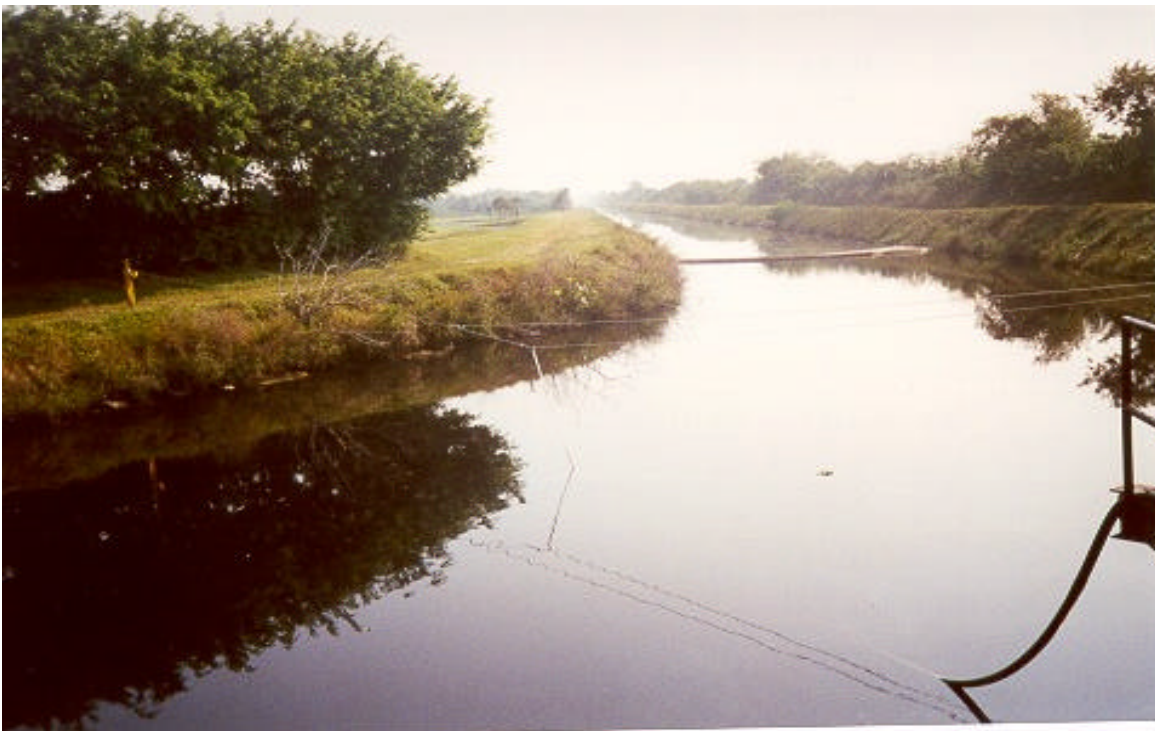
FIGURES 4a and 4b. PILOT UNIT INTAKE STRUCTURE IN UPSTREAM CANAL May-01
