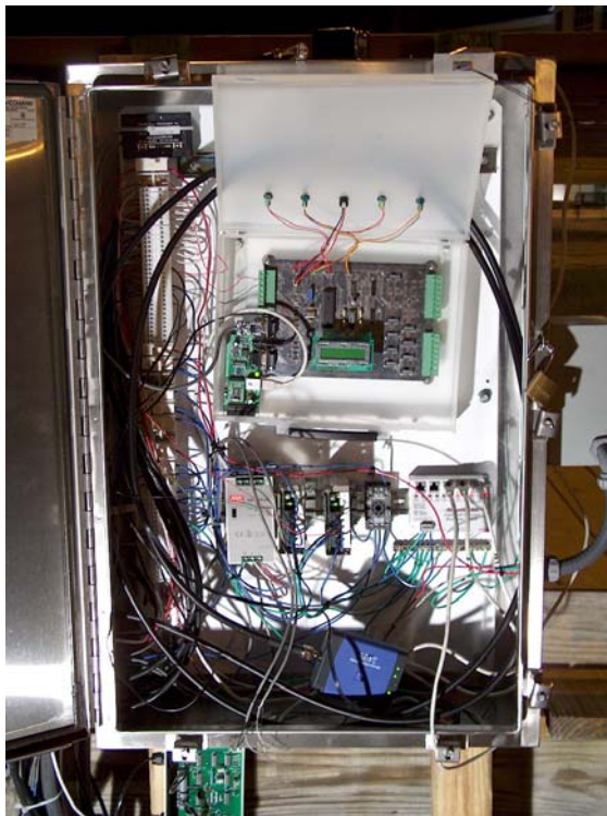
Figure 2: MCU & PLC Interface
