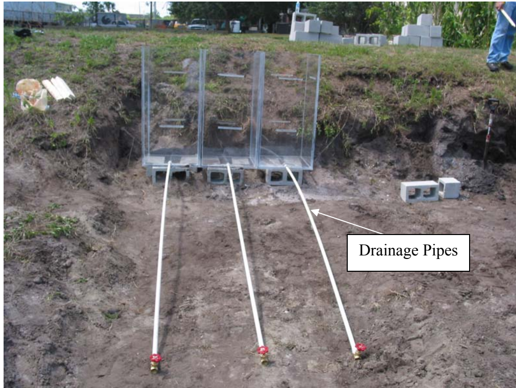
Figure 9 – Chambers before backfill
