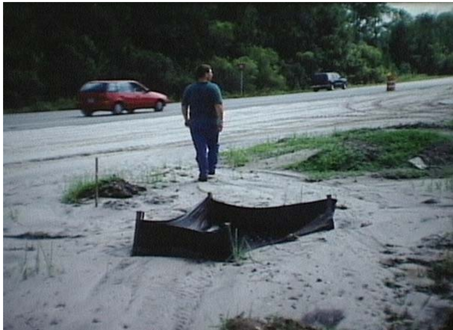
Temporary filter system surrounding storm drain inlets.
