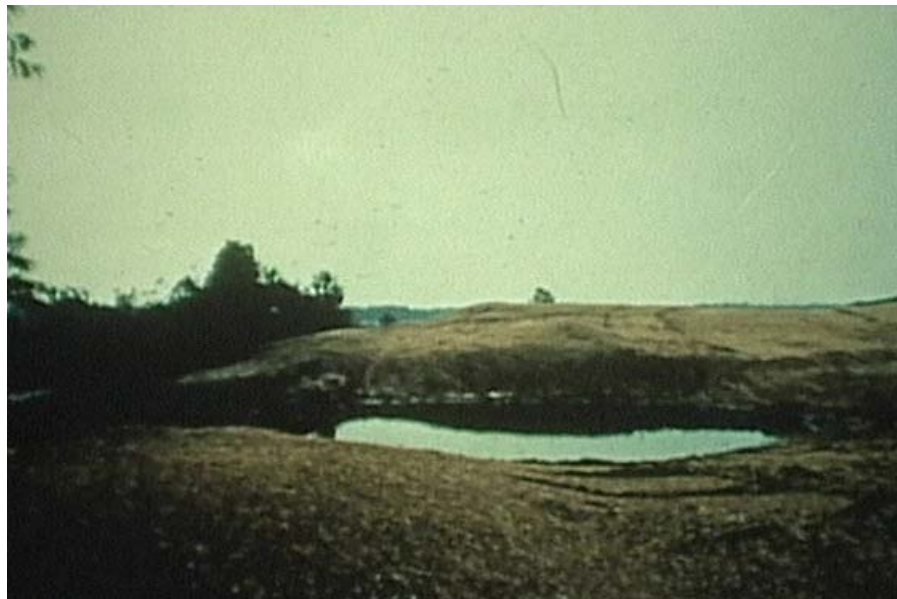
Small temporary ponding area formed by constructing an earthen embankment with an outlet across a swale.
