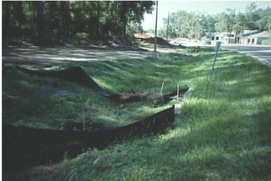
Small temporary dams constructed across a swale or stormwater conveyance channel.
