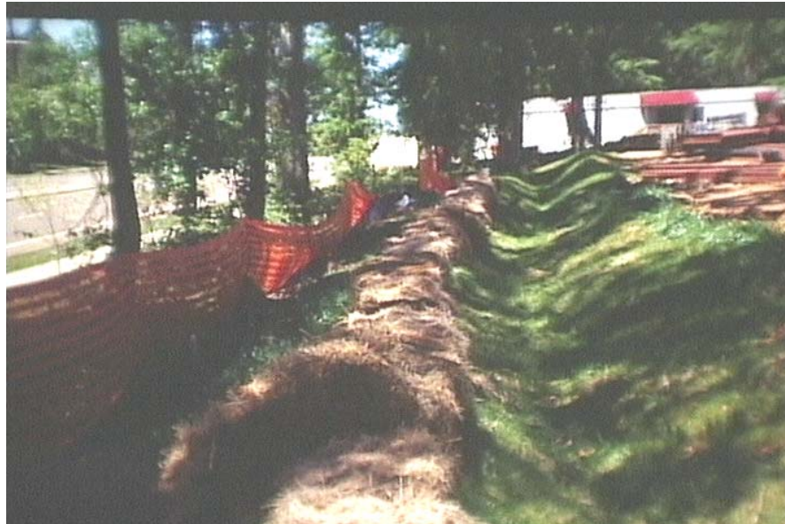
Diversions composed of compacted earthen ridges.
