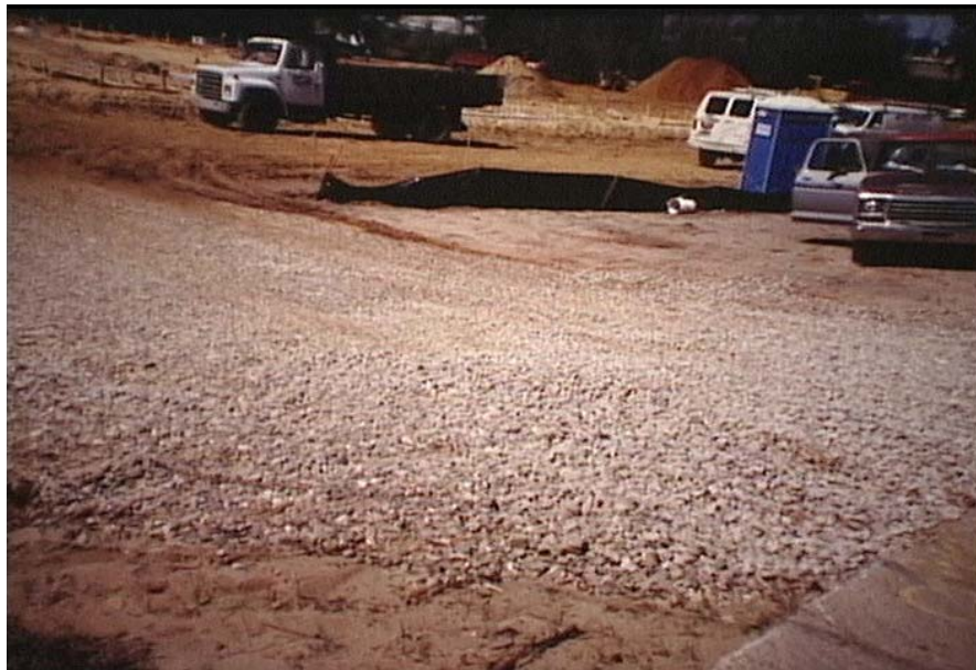
Stone stabilized pad located at vehicular exits and entrances on a construction site.
