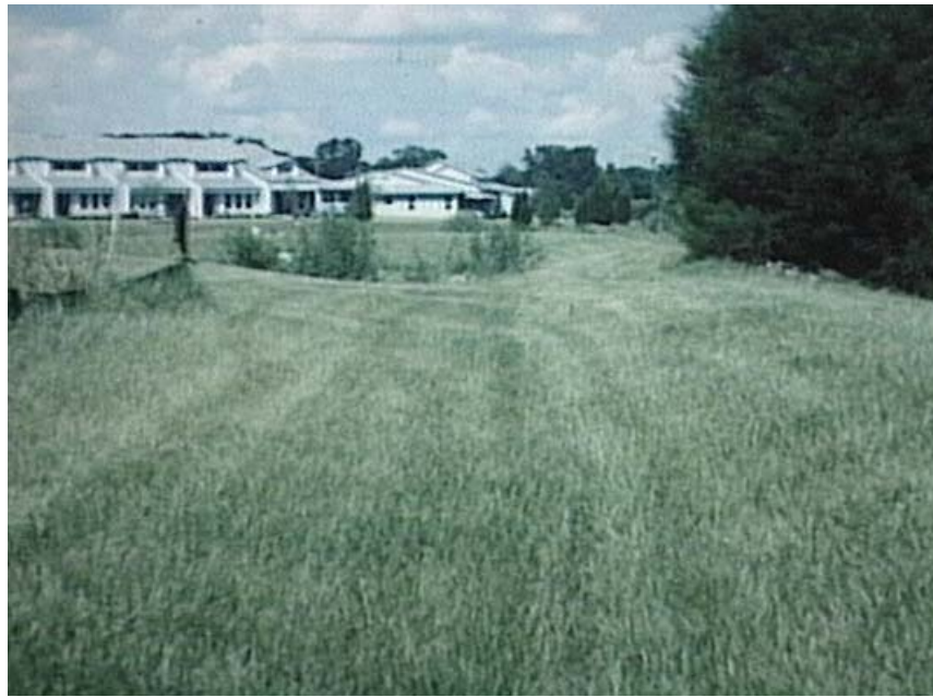
Permanent designed waterway to transport excess stormwater runoff away from developing area.
