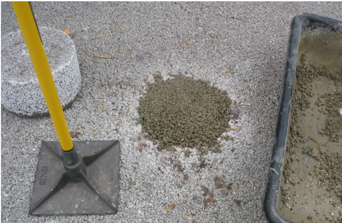
Figure 11: Repair of Concrete Core Area
