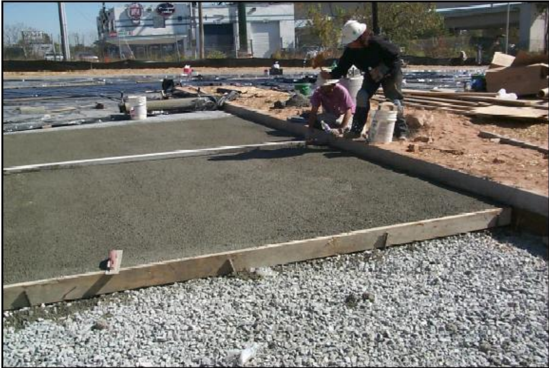
Figure 2: Typical Porous Concrete Installation
