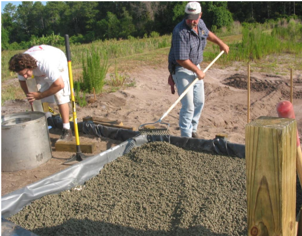
Figure 3: Stormwater Academy Porous Concrete Test Cell Installation
