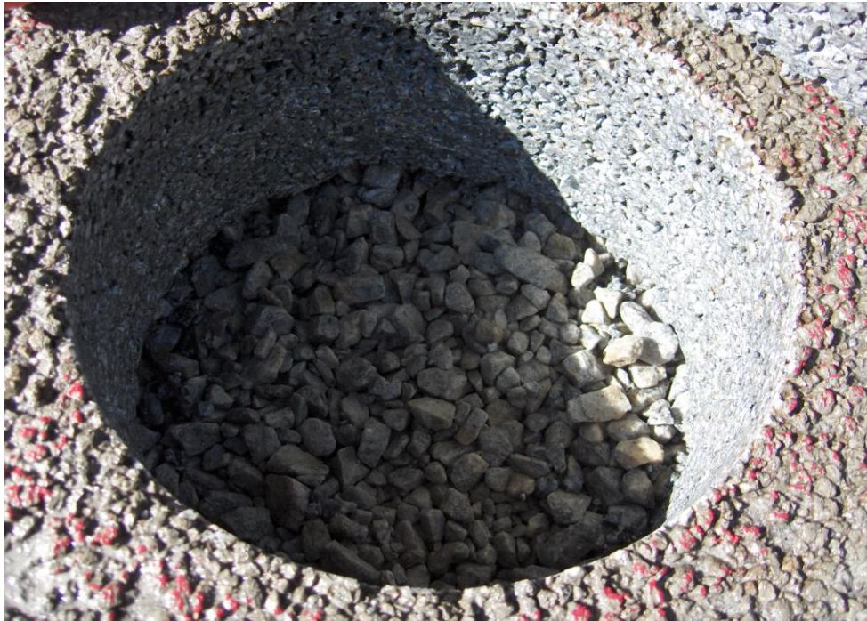
Figure 27: Southface Institute Gravel Subbase
